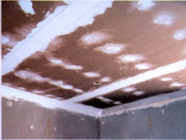
A 9.5 Rhinoboard ceiling with skimmed joints.
